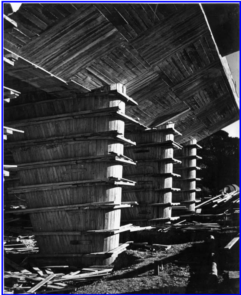
Figure 22 Le Corbusier, Unité d'Habitation, construction view of the pilotis, shuttering, and checkerboard canopy on the south side, ca. 15 November 1948 (Fondation Le Corbusier, Paris, FLC L1.13.81; © F.L.C./ADAGP, Paris/Artists Rights Society [ARS], New York 2014).
